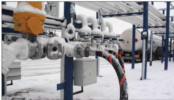
The TODO® SAFETY BREAK AWAY coupling are designed to eliminate spillage and damage associated with drive / pull away incidents. Offer exceptionally high flow capacity for their size.
