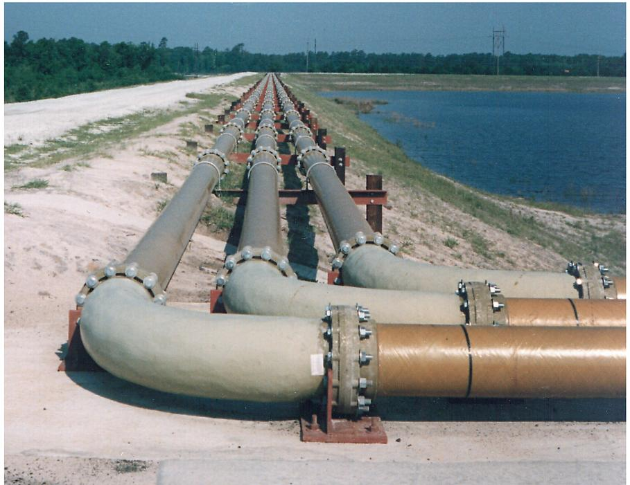
*Ninety degree sweep elbows lined with ceramic tiles are one of the fittings choices you have when designing a complete CERAM CORE piping system.*
