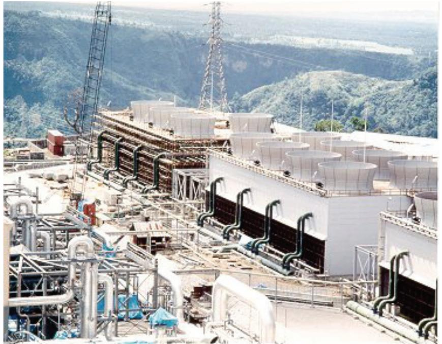
*F-CHEM custom piping is supplied for condensed steam cooling tower supply and return lines at geothermal power plant.*
