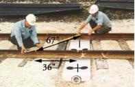
diagonally to opposite rail. The two marks on the rail must be lined up with center of cross drain. Contact Century if the track is not tangent.
