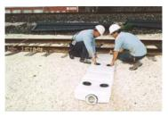
6. Align the center of the cross drain with the center line of the track. The HDPE Enviropan® is
