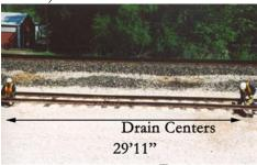
3. Space crossties at locations of the cross drains to allow for 24" clearance to accept the cross drain.
