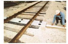
10. Ballast shoulders should extend 4'0" from the outside ball of rail on both sides of track (see diagram below).
