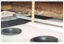
make sure that the center of the cross drain is still centered with the center line of the track (tangent  $28 \ 1/4$ ") and the cross drain is square to the rail.
